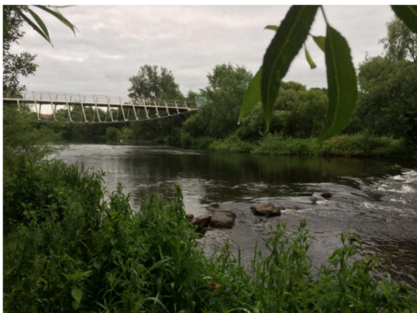
Living Bridge University Campus Limerick
